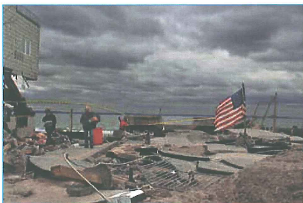
Serious damage to the buildings at the Seagate neighbourhood due to impact from Hurricane Sandy in Brooklyn, New York, U.S., on Thursday, 1 November 2012.
